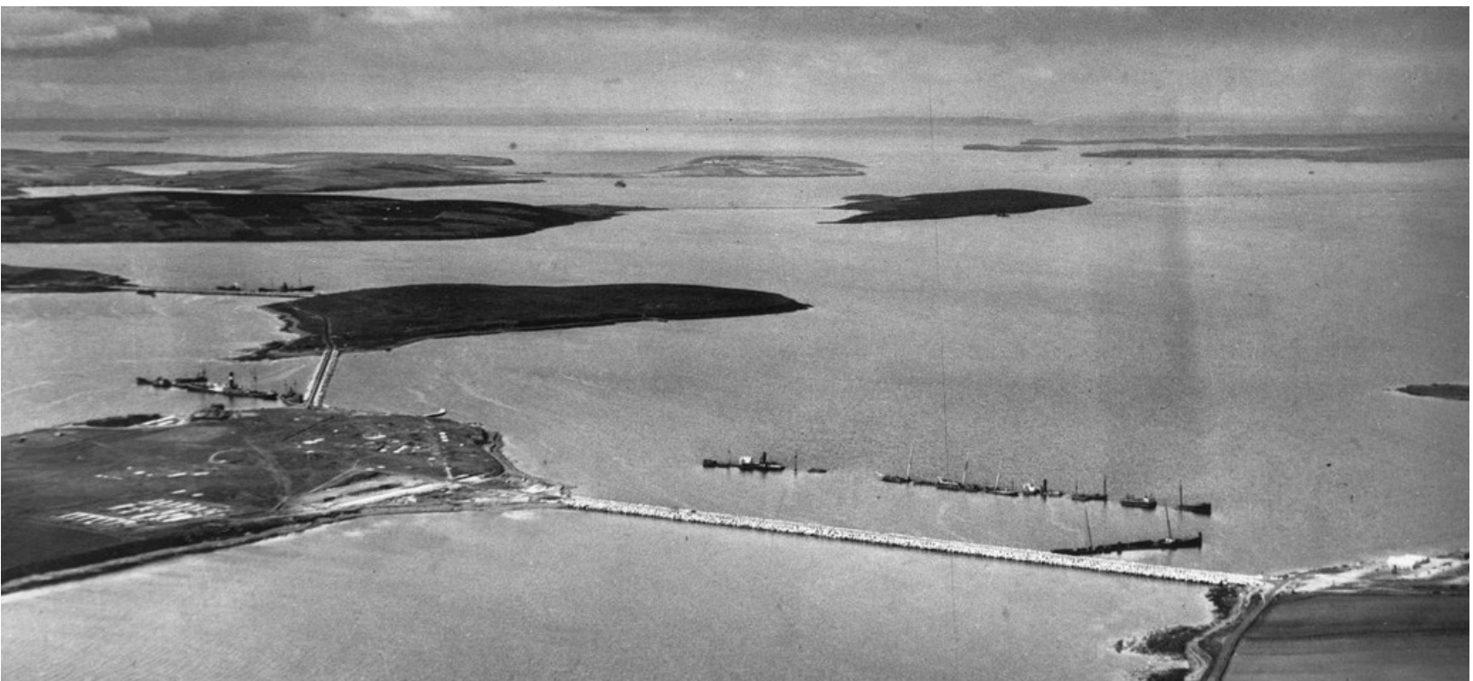
Churchill Barrier. Around 350 British workmen and nearly 1300 Italian prisoners of war captured in North Africa built the four causeways to protect military vessels at Scapa Flow.
