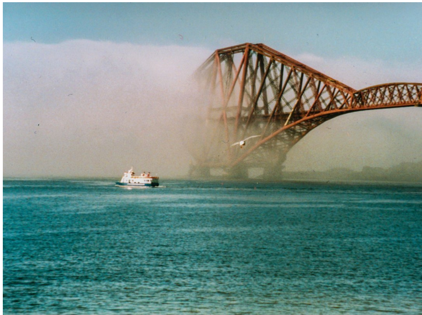
Forth Rail Bridge taken from South Queensferry Pier.
