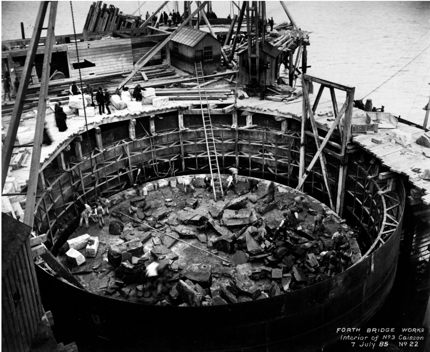
Construction of Caissons, 1885 – South Queensferry.
